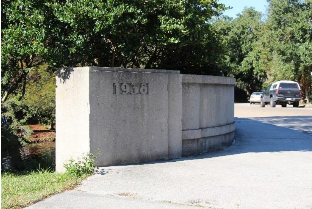
Character-defining Feature Photo 3: Design of reinforced-concrete superstructure with integrated curved wing walls and aesthetic treatment seen in bold font in Art Deco style letters in the concrete endposts and crowned parapets/railings (Recall No. 102234 shown).
