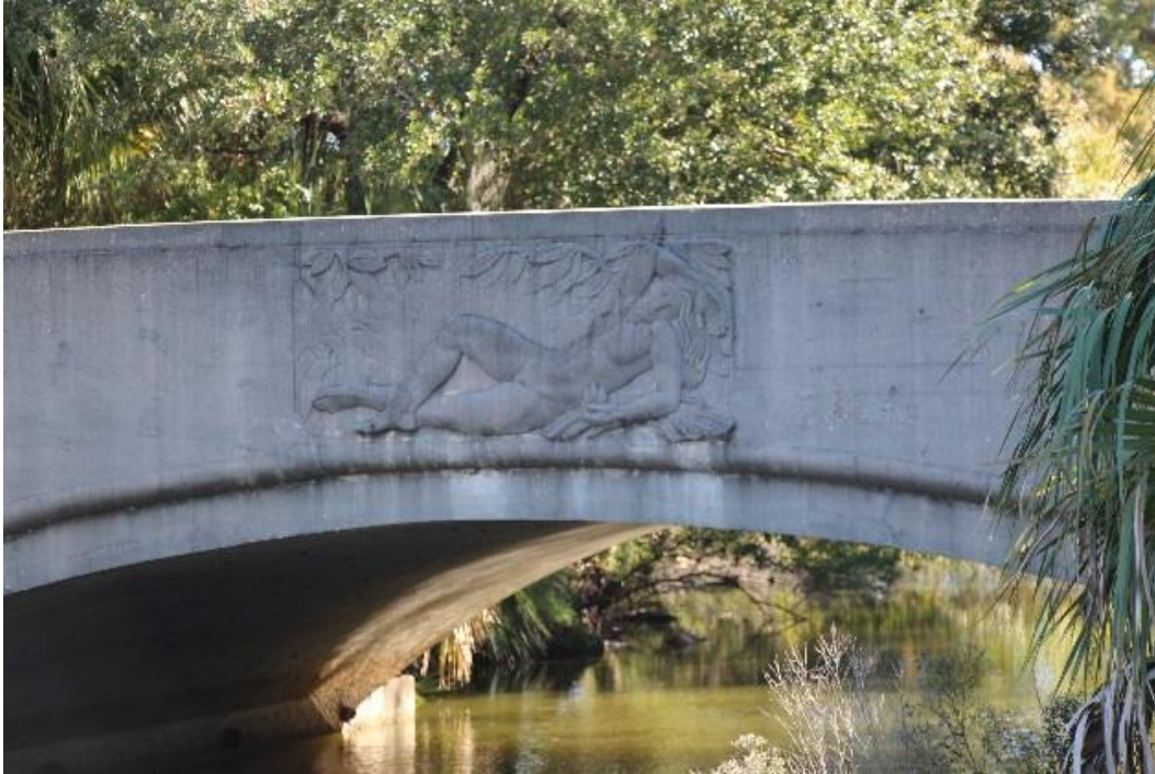
Character-defining Feature Photo 11: Aesthetic treatment seen in bas-relief sculptures (Recall No. 102235 shown).
