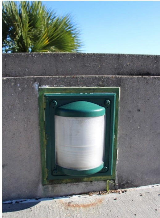
Character-defining Feature Photo 9: Aesthetic treatment seen in integrated lighting and beveled parapets/railings (Recall No. 102233 shown).
