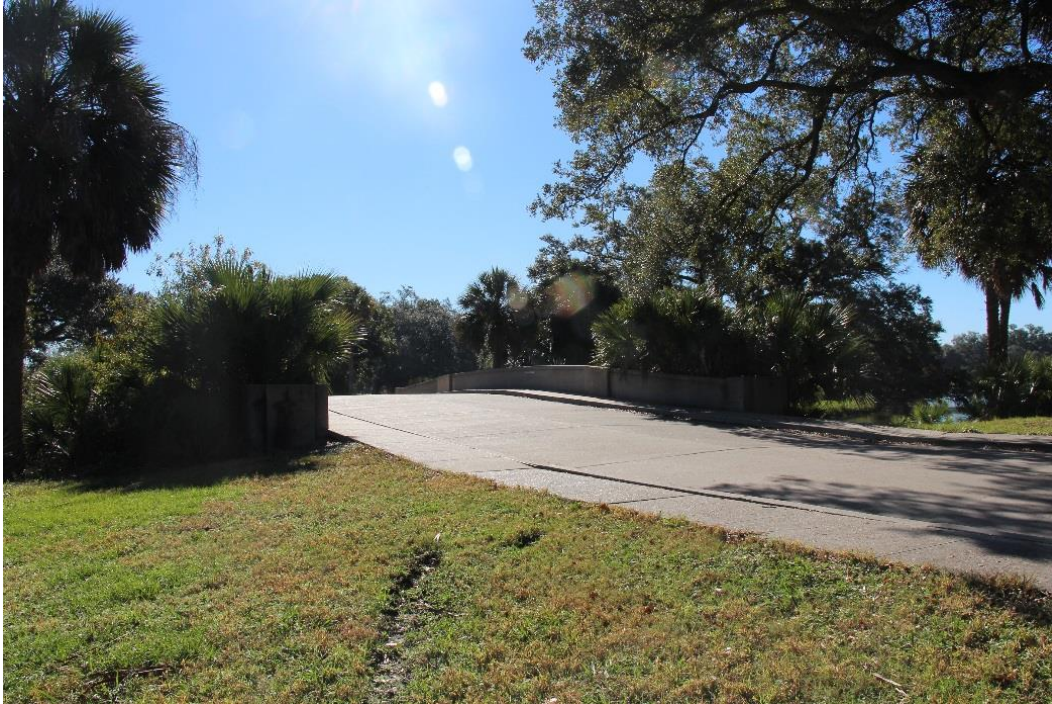
Condition Photo 20: Unsealed joints in concrete sidewalk on Recall No. 102236; settlement at curb line.
